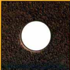
Hole drilled with diamond core
